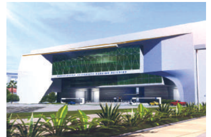
Torpark system, Thailand - 840 cars
